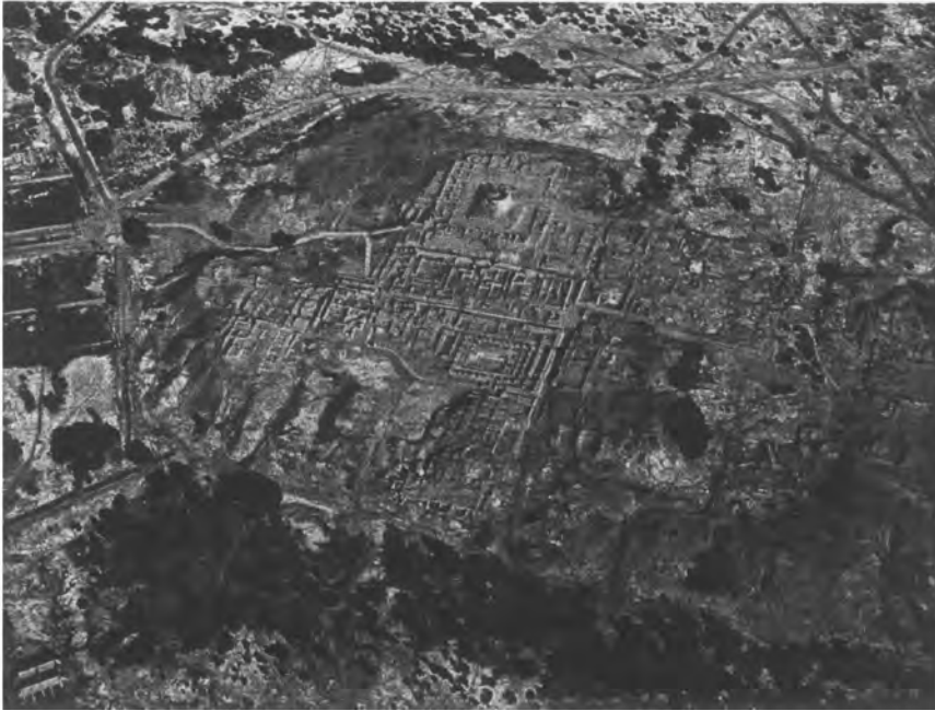
Figure 4 The 'Citadel' sector was excavated by Sir Mortimer Wheeler. In the background is the Buddhist stūpa and in front of this are the two large structures discovered by Wheeler which he named the Granary and the Great Bath. Wheeler thought that wagons loaded with grain entered the citadel from the west and were unloaded in front of the Granary. Recent research has shown, however, that the upper section of the Granary does not date from the same period as the lower section which is older. It is thus probable that Wheeler's theory is incorrect and that the building had a different function. (Photo: Research Project Mohenjo-Daro).
