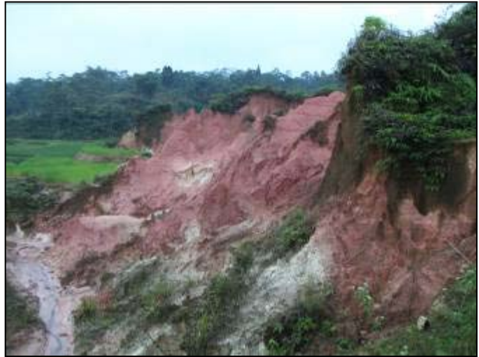
Figure 19. Example of extreme erosion in GHNP.
