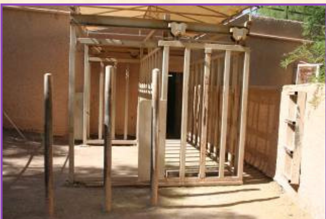
Chute before modifications
