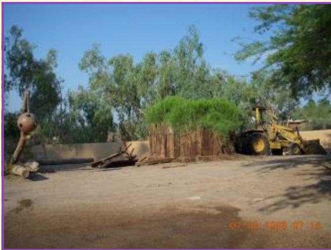
Removal of planter
