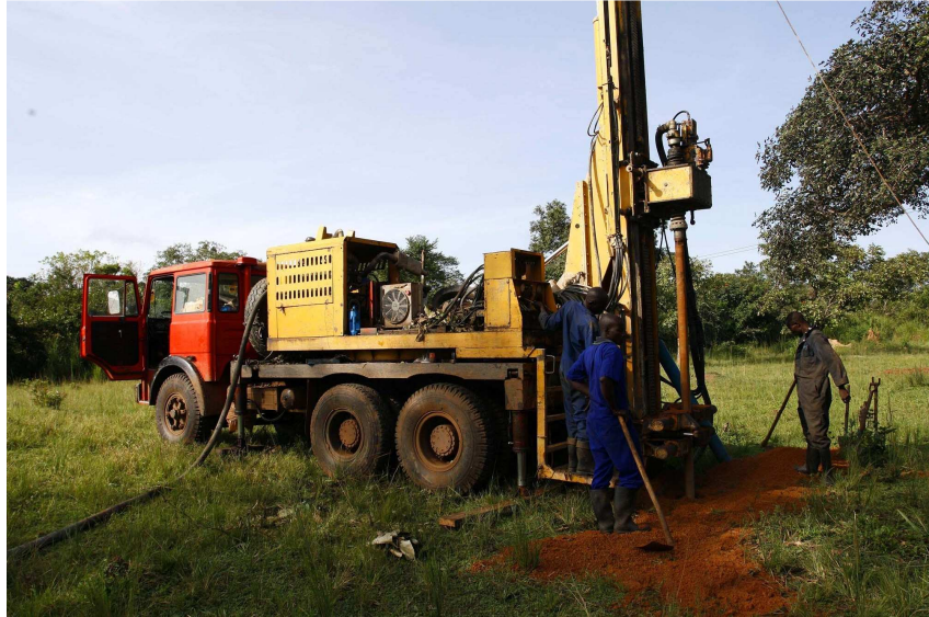
Waterhole construction
