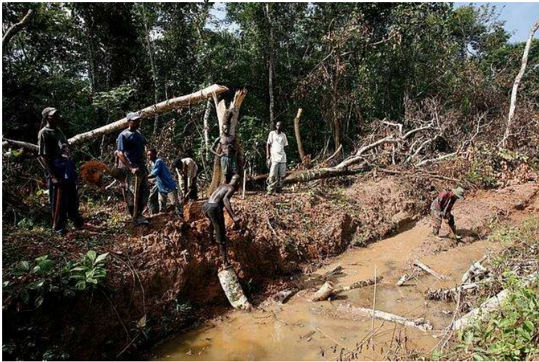
Work on the road to Faradje
