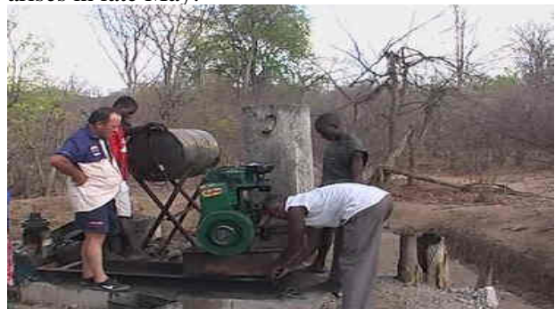
Johnny overseeing repairs to a pump.
