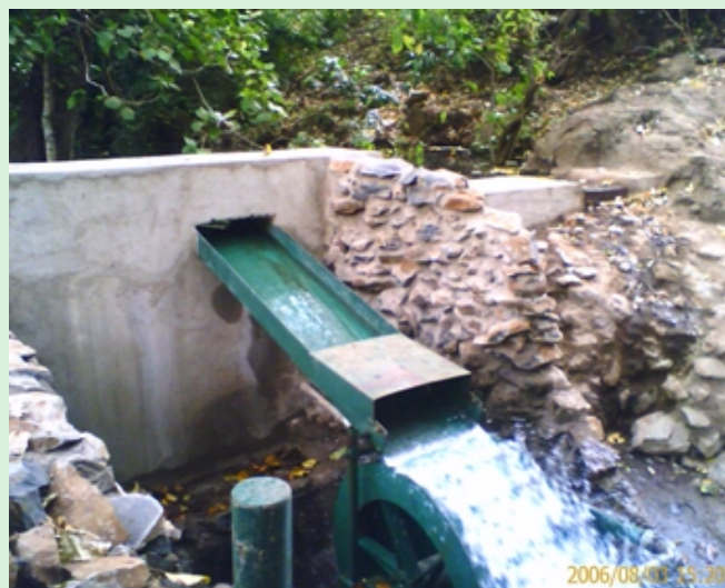
Mkuu water project under construction
