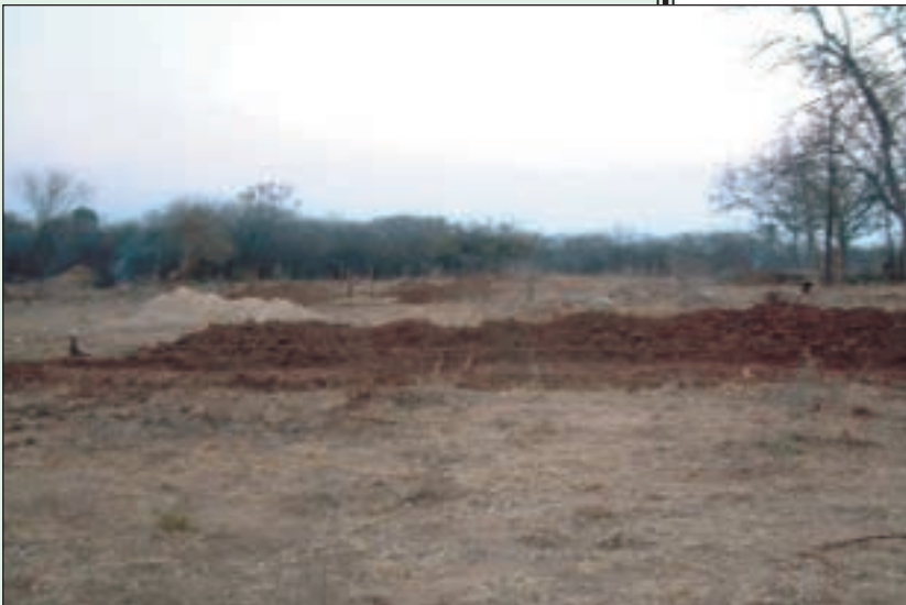
Completed site clearance & preliminary excavation works
