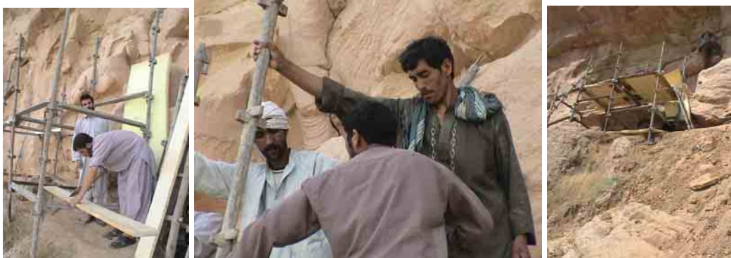
Building the platform.
