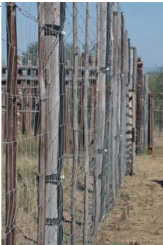
Wholly electrified Bonnox wire mesh fencing on wooden posts with used polyurethane piping and (white) Meps bobbin insulators.
